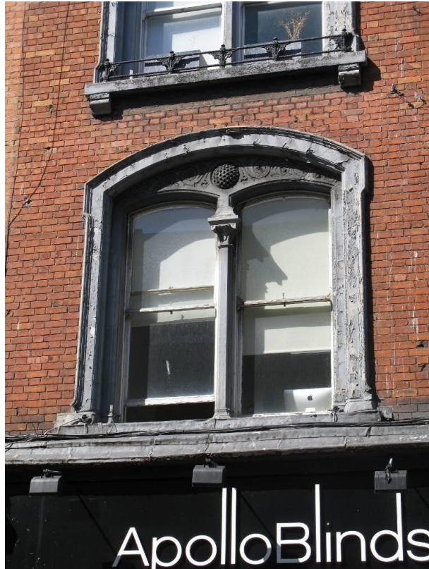
Paired first floor timber sash windows
