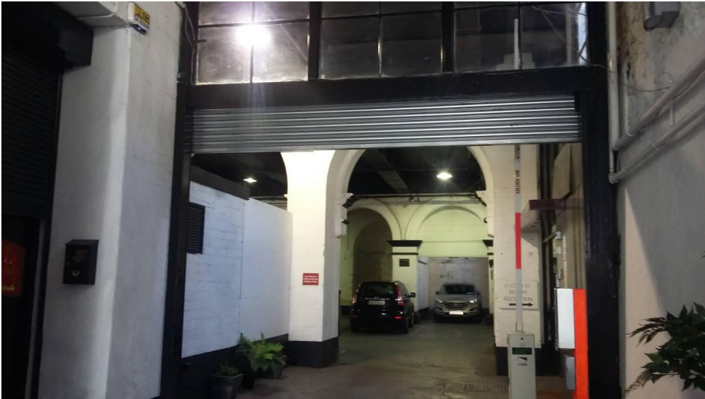
View through from 133 Capel Street through to 133A -133B Capel Street
