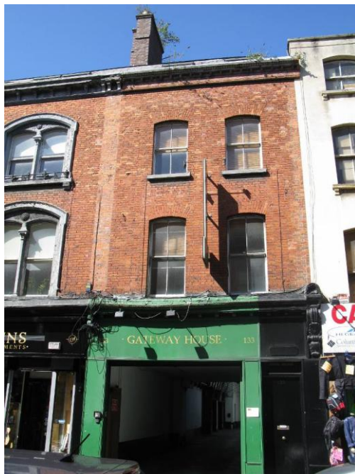
Carriageway through 133 Capel Street
